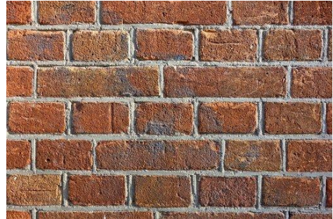
A brick wall
